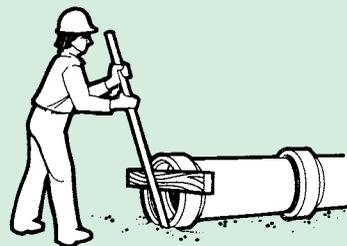
Wedge bar against a wood block placed horizontally across the bell end of the pipe. Pressure on the bar pushes the pipe into the home position.
